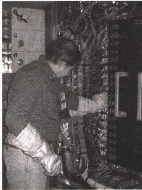
Hold On! —IEEE member Ken Innes (left) attempts to grasp a power connector while wearing bulky astronaut gloves. The power unit is identical to a replacement unit installed in HST and was used in the High Bay Clean Room to train astronauts for the repair mission. Goddard's 120-foot-diameter centrifuge (above) can accelerate a 2.5 ton payload up to 30 Gs, well beyond the force experienced during a launch.
